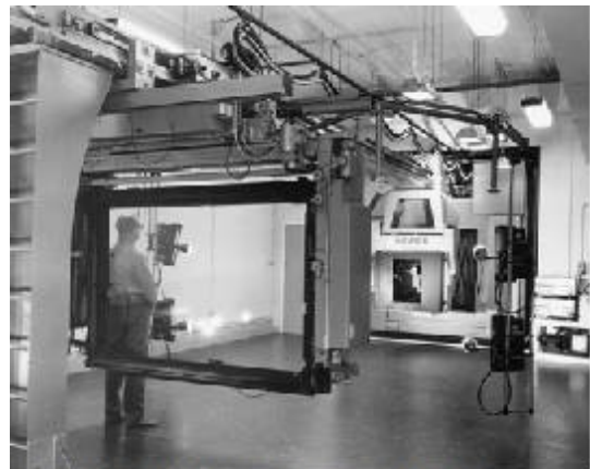
Klimsch 27042 installation in the Land Administration Building
