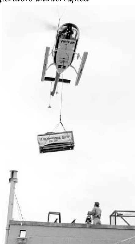
A local TV station helicopter was recruited to lower the air conditioning unit onto LAB
